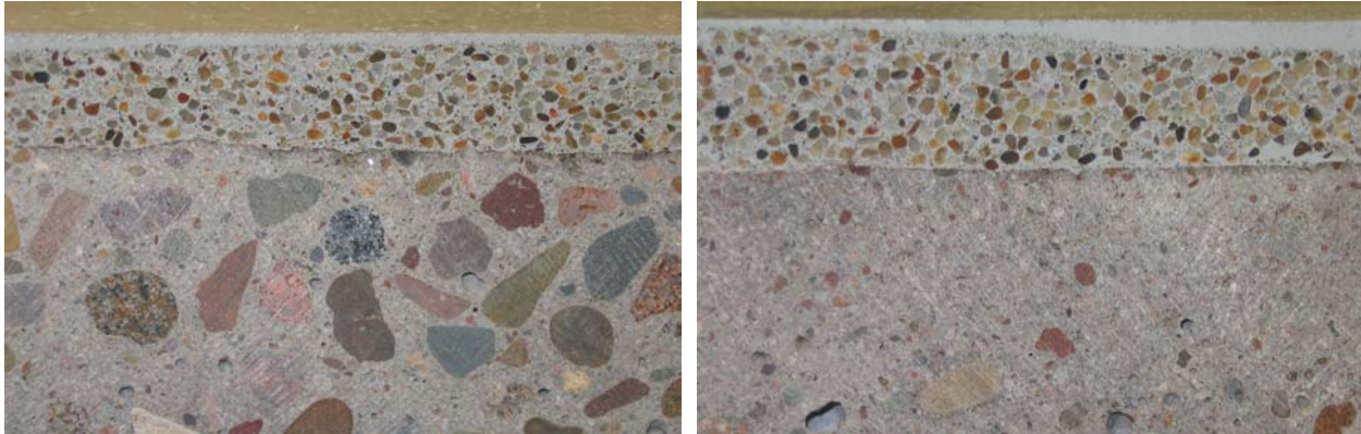
Figure 4. Thermal compatibility slabs after thermal cycling (Left-near center of test slab, Right-near edge of test slab)
